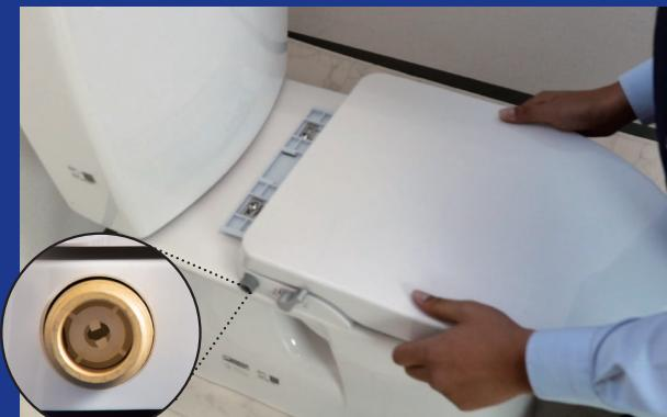
※SG-002の接続部は金属製／SG-002 connecting part is made by metal
